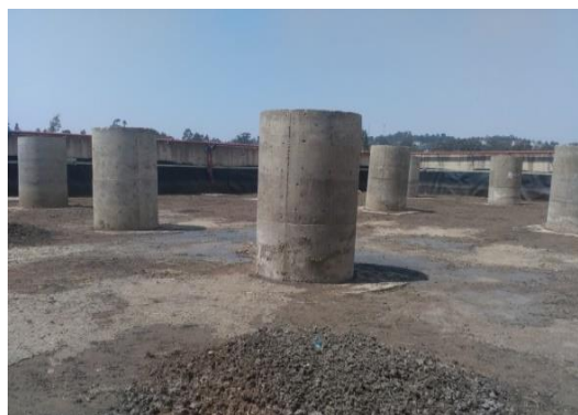
Figure 3: The drying beds of the sludge
