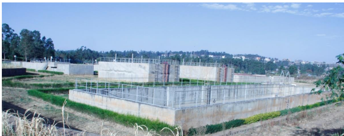
Figure 1: Debre Markos University waste treatment plant
